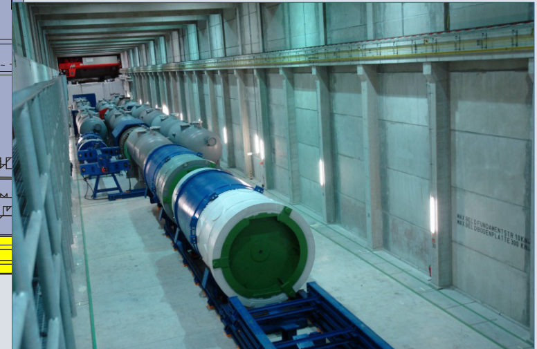
Removed vessels und steam generators
